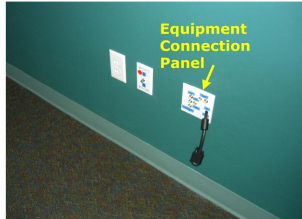
Equipment Panel Connections
